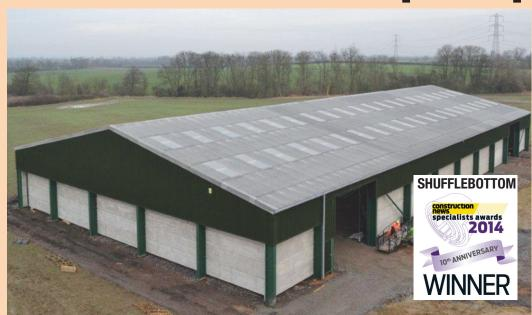
The substantial Shufflebottom grain store on B&J Wiles & Son's Brinvale Farm at Long Clawson near Melton Mowbray in Leicestershire, stretches for 200 feet and is 100 feet wide. Concrete panels 180mm thick and 4 metres high allow for three openings, two of which have
